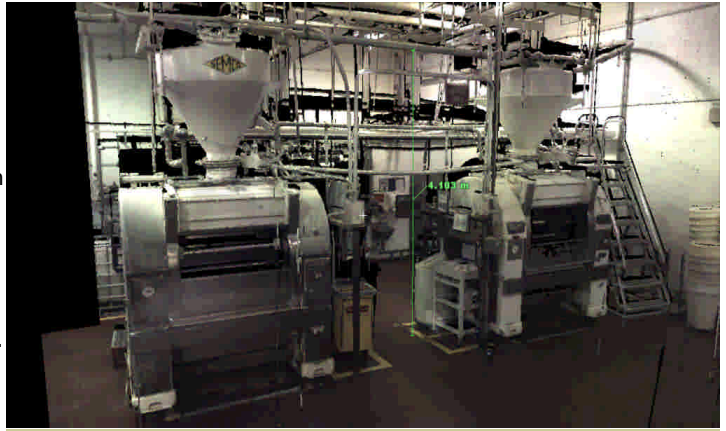
Point Cloud data showing clearance dimensions to pipe.
